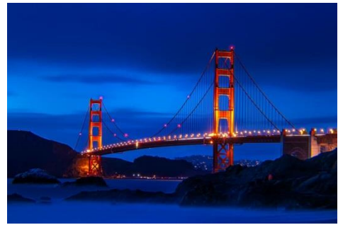
The Golden Gate Bridge from the Marin Headlands
